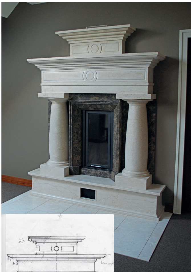
Hand-made portal for a fireplace, drawing and the realisation, combination of two types of marble (220 cm)
